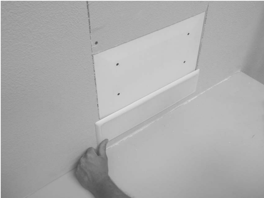
Figure 23: Finished Grille Installation
