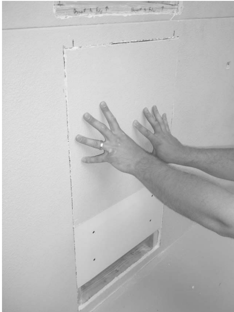
Figure 48: Drywall Installation
