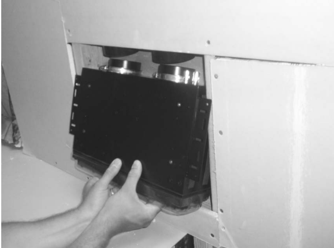
Figure 7: Driver Module Installation
