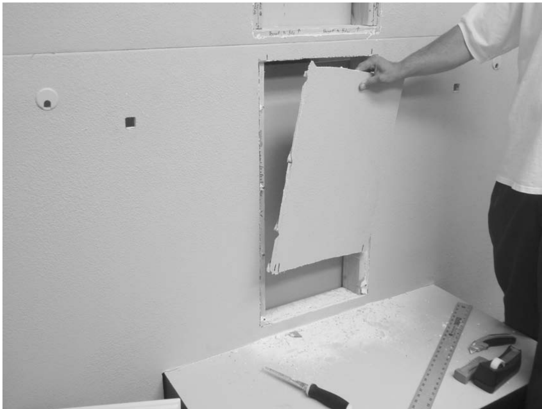
Figures 26a and 26b: Drywall Removal
