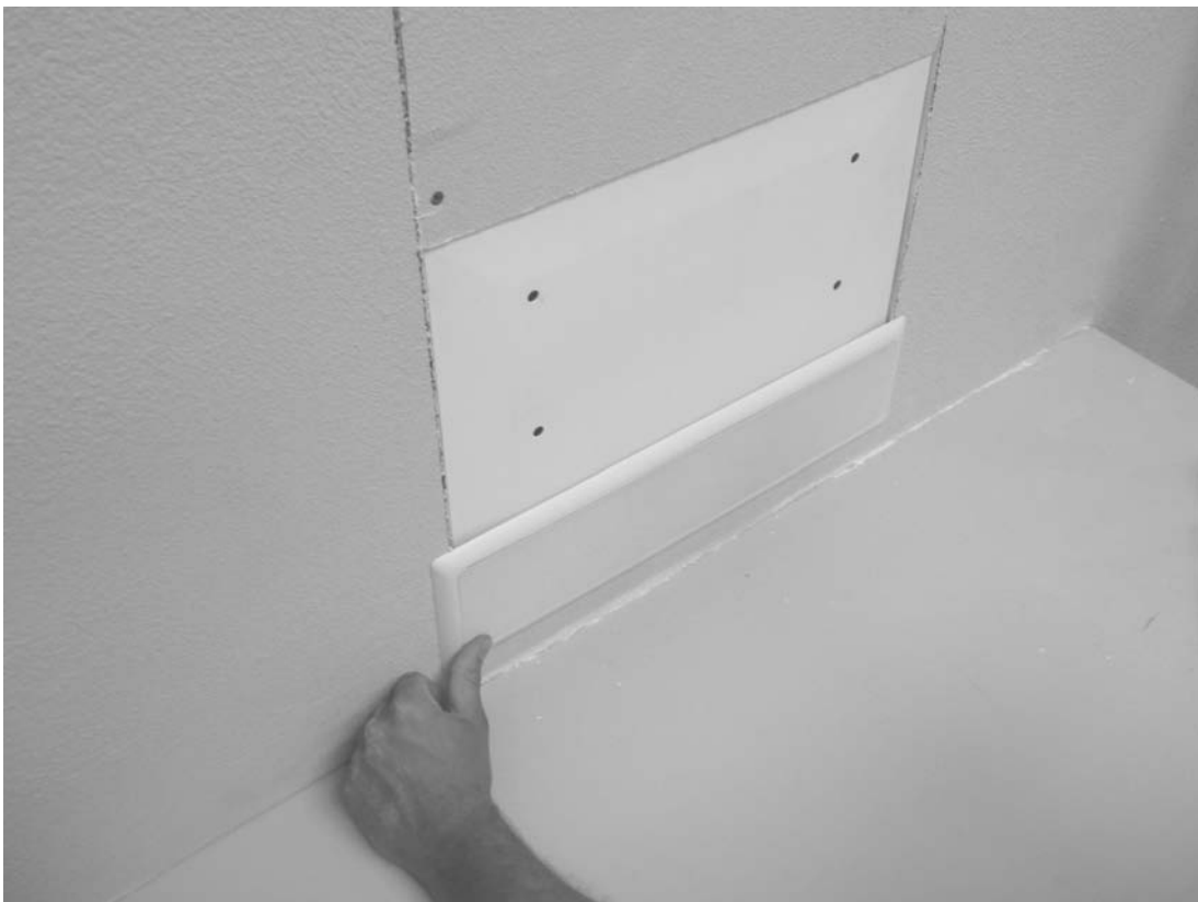
Figure 37: Finished Grille Installation
