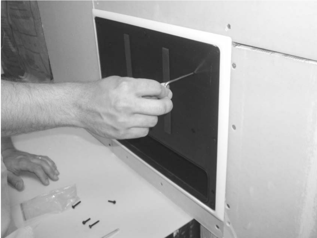
Figure 9: Grille Frame Installation
