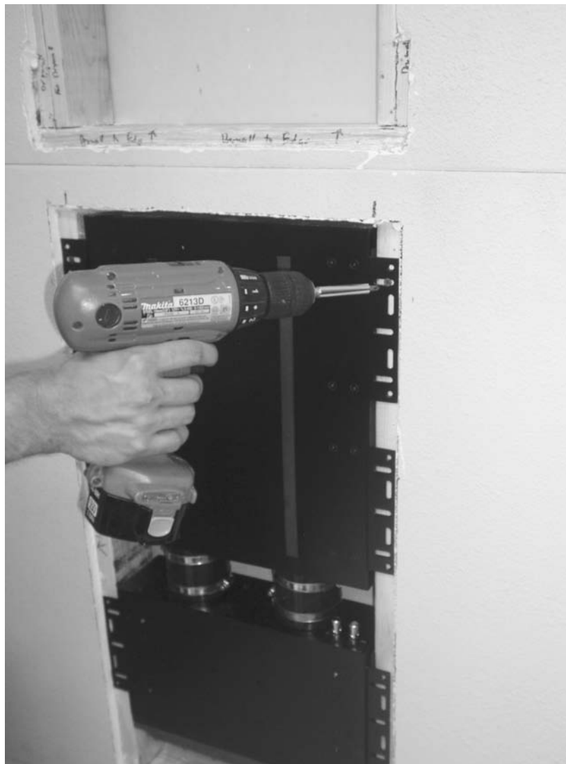
Figure 31: Secure Subwoofer
