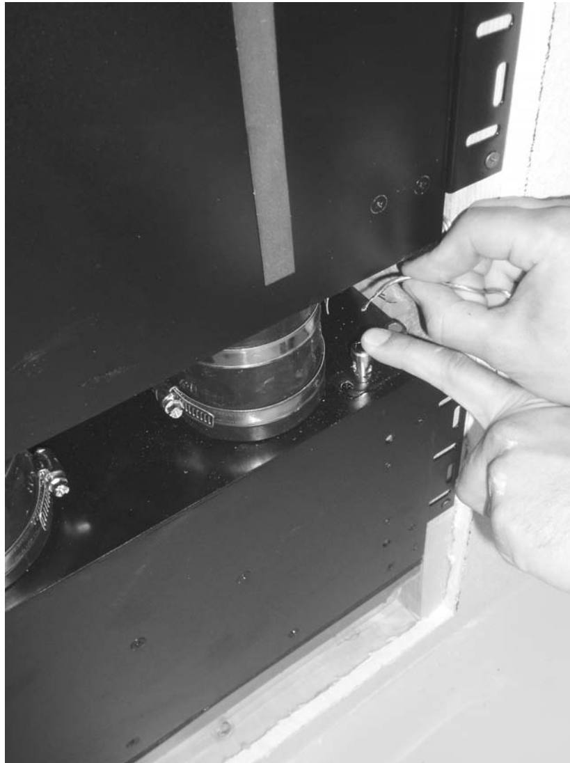
Figure 17: Speaker Wire Installation
