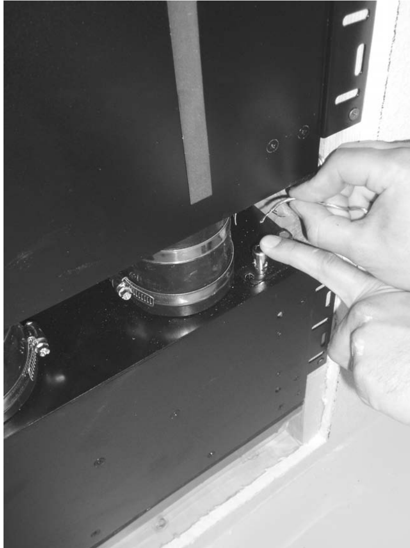
Figure 46: Speaker Wire Installation
