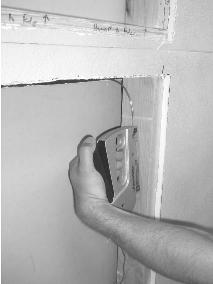
Figure 41: Speaker Wire Installation
