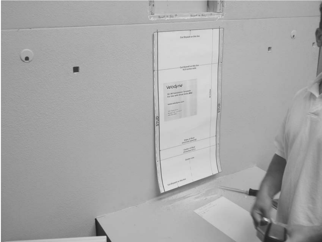
Figure 25: Cut Out Drywall Per Template
