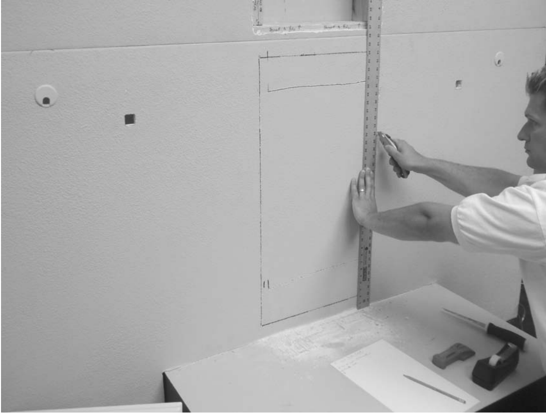
Figures 26a and 26b: Drywall Removal
