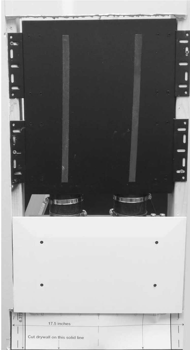
Figure 19: Template Place Holder Installation
