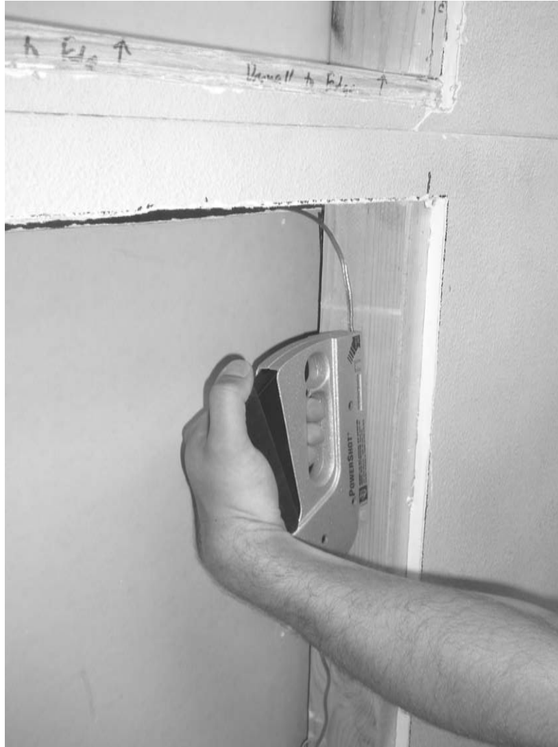
Figure 27: Speaker Wire Installation
