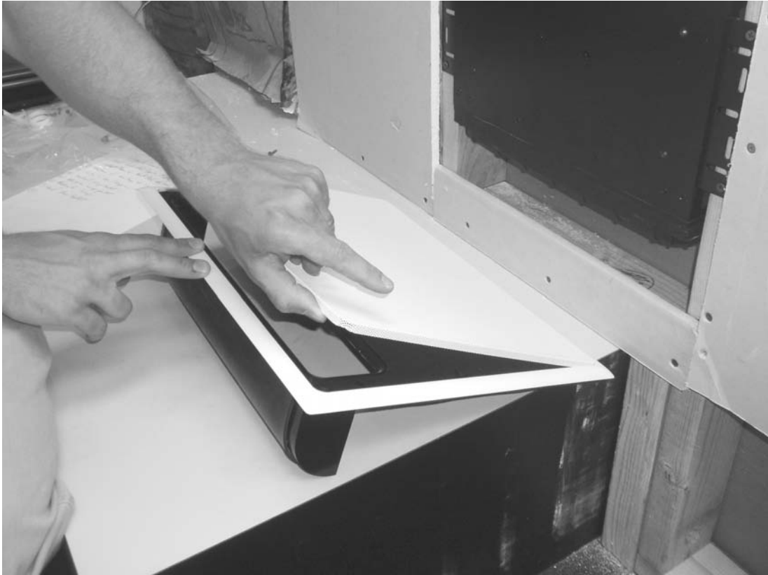
Figure 49: Metal Grille Insert Removal
