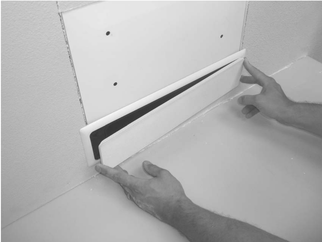
Figure 22: Metal Insert Installation
