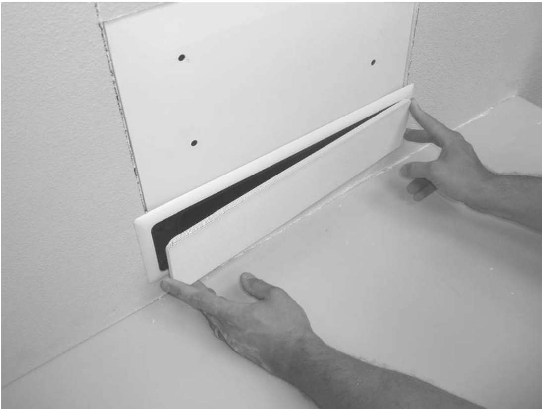
Figure 36: Metal Insert Installation
