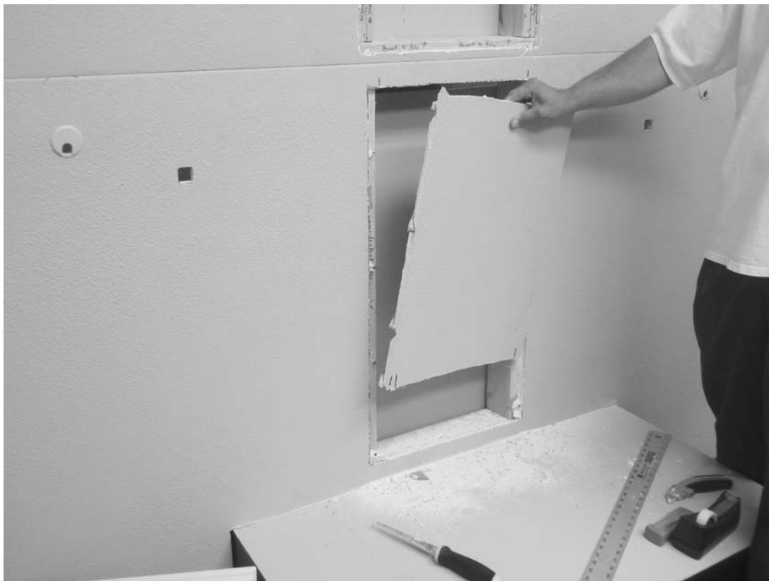
Figures 40a and 40b: Drywall Removal
