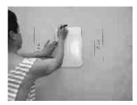
) Using a drywall saw, cut out the opening.
