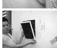
) Align the speaker in position, and tighten the screws evenly to secure the unit.
